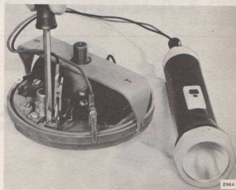
Figure 4-20. Adjusting Breaker Points
